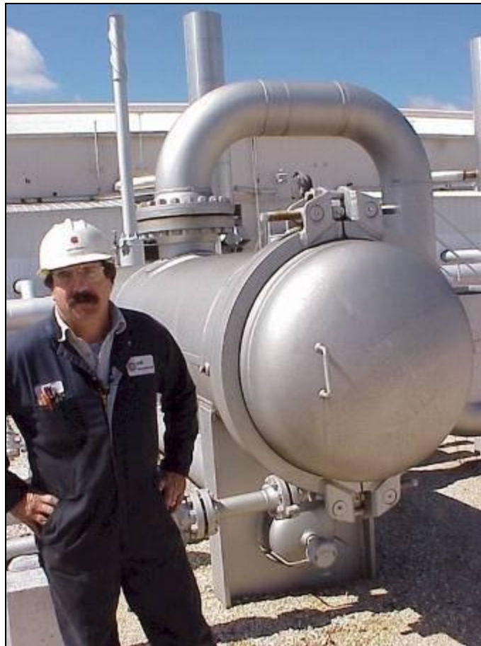
This Full-Opening Hinged Closure Facilitates Access to the Filter Elements
